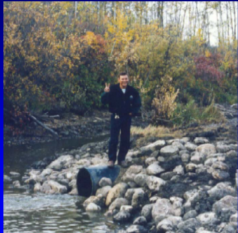
Danny Fisher, Chairman during installation of the pipeline
