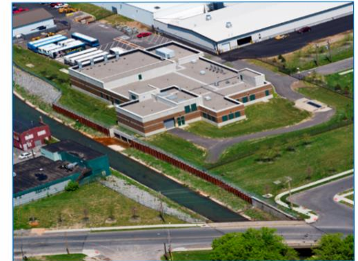
Midland Avenue Sewage Treatment Plant
