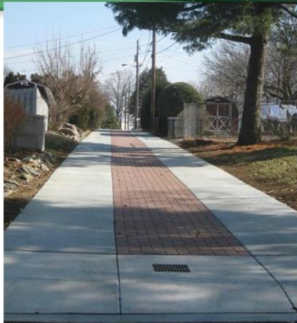
Green alley retrofit (permeable pavers with infiltration trench) ~$22.40/SF
